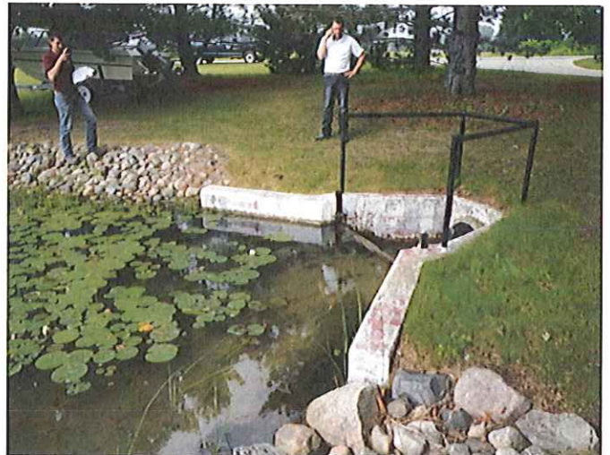
Inlet Structure-East Side
