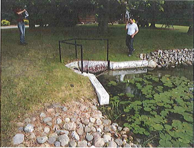
Inlet Structure-West Side
