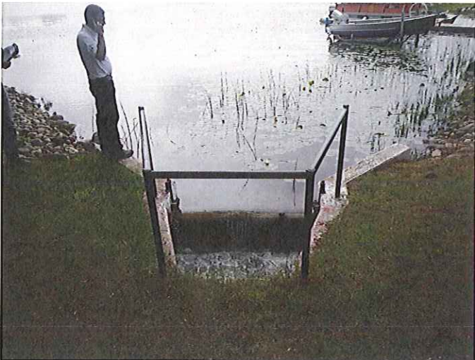
Inlet Structure Upstream
